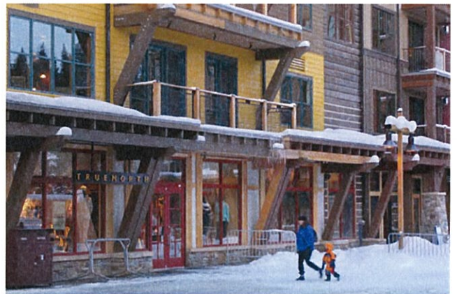
Image 17. Protruding overhead canopies create interesting architectural façades and provide protection from falling snow.
