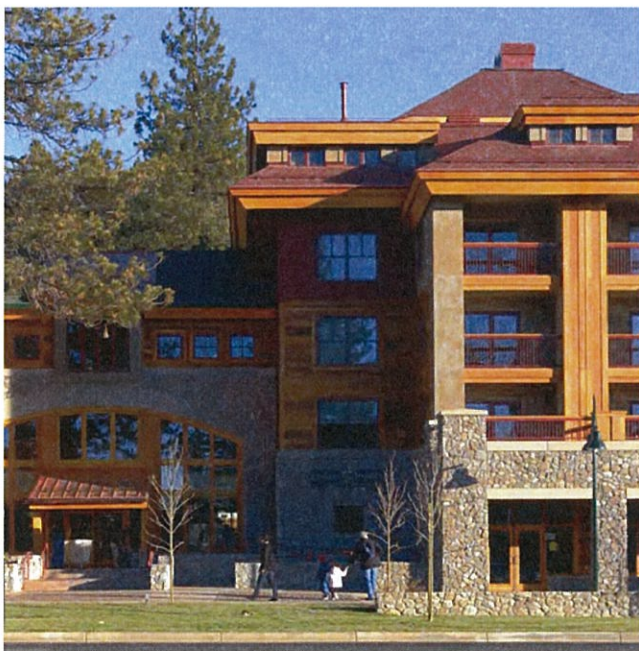
Image 28. Varying wall planes reduces the visual scale of a structure and helps to highlight interesting building features.
