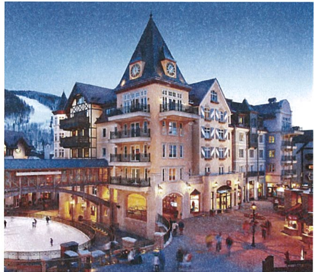
Image 31. Distinctive roof lines are created with roof forms and building heights that vary.
